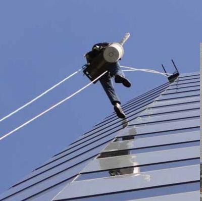
The Rack is a one of a kind fall protection rated anchor point system designed specifically for window washers using bosun chairs. The Rack, invented by an industry expert, was designed to provide a much safer means of accessing the leading edge and descending during window cleaning operations.
